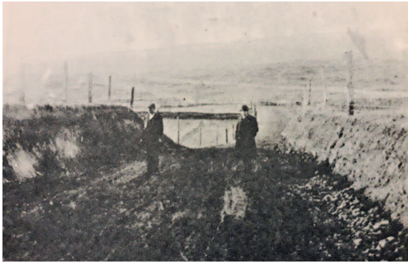
Mr. Benjamin Murrow with Mr. Tom Higgins during the construction of Buenos Ayres Drive, c.1915. This picture was taken from the top of the present Buenos Ayres Hill. (Photograph courtesy of John C. Mc Ternan, At the Foot of Knocknarea)
