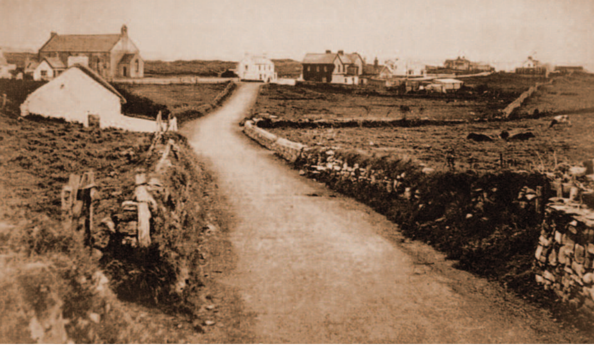
A photograph of St. Patrick's Church taken from the present day Burma Road. Thady Higgin's cottage is on the left hand side of what was locally referred to as Thady's Lane. Thomas Mannion's house is on the western side of the church and St. Patrick's Hotel directly opposite.
